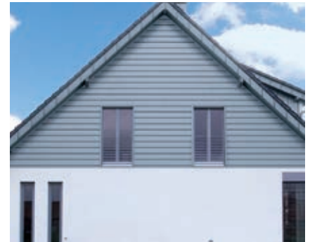
Gable cladding at residential building
